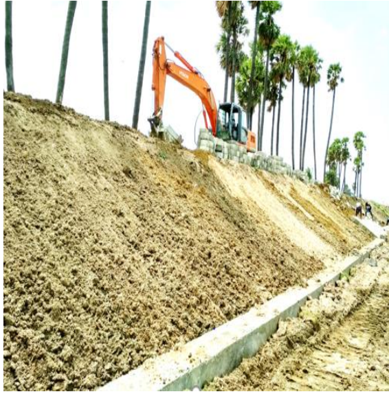
Figure 11: Casting and Fixing of CC Blocks
