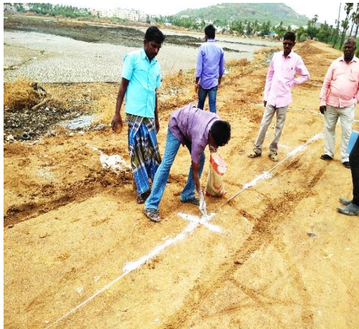
Figure 5: Construction of Regulator in Pallavaram Lake
