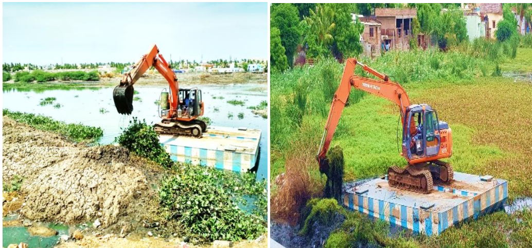
Figure 6: Removal of Floating Materials in Pallavaram Tank
